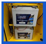
Release the retaining bars on the battery storage and withdraw one battery at a time. Remove the terminal cables, paying close attention to their orientation. Place the charged batteries back into the cabinet and reconnect as previous.
